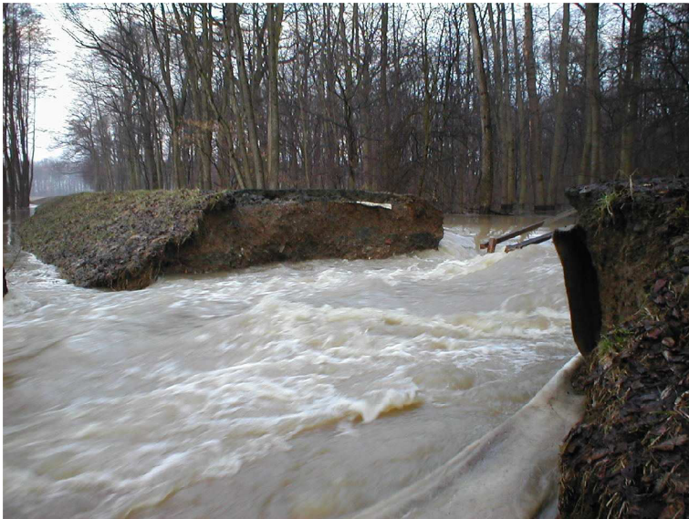
Fig. 6.7 Fourth phase: dike collapse
