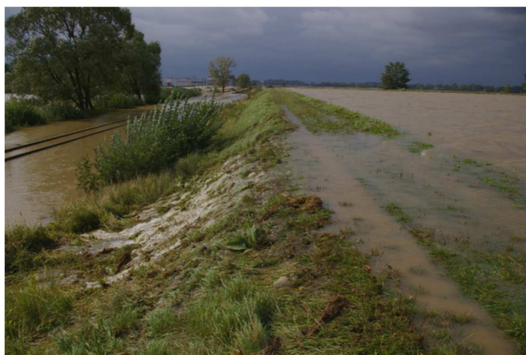
Fig. 6.5 Second phase: overtopping - no erosion
