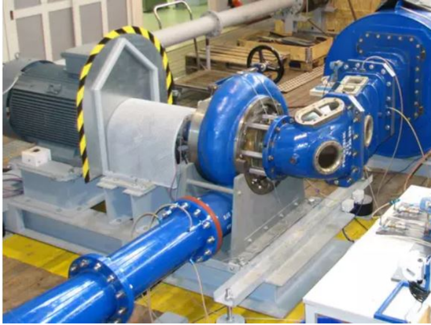
Figure 3: Installation site of PAT [3]
