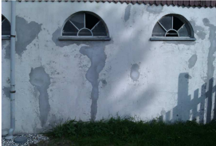
Fig. 60 The reference old stable for the pilot test.
