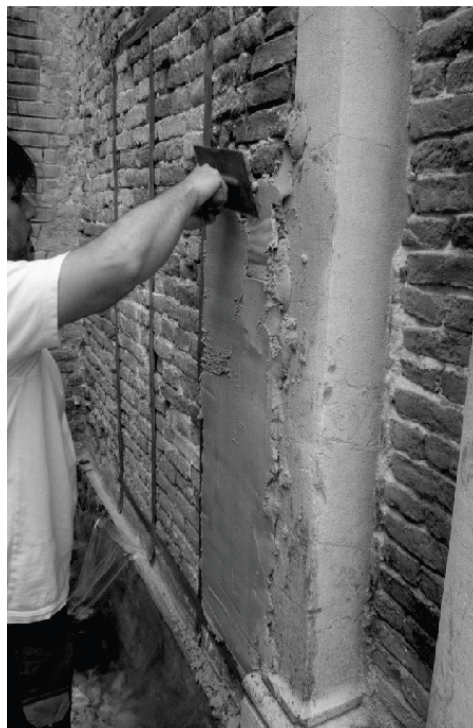
Fig. 13 Application of poultice on the brickwork. [30]
