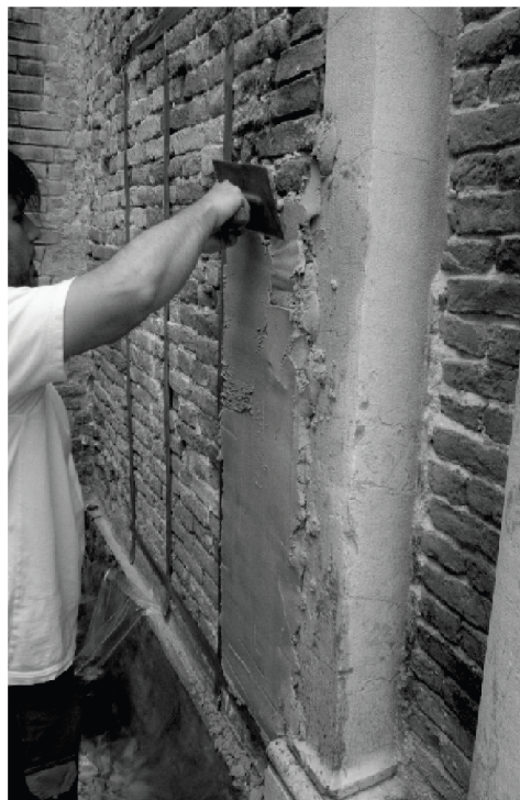
Fig. 13 Application of poultice on the brickwork. [30]
