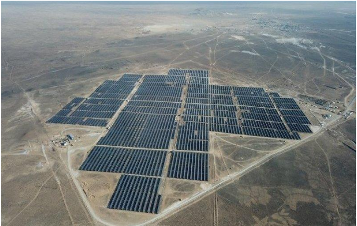
Figure 8. Source Tengri News https://tengrinews.kz/progress/solnechnaya-elektrostantsiya-gulshat-otkryita-karagandinskoy-367926/
