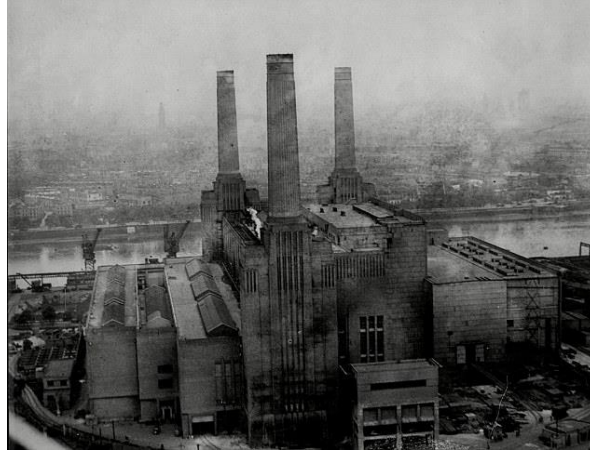
Figure 1 – Battersea Power Station, London (photo courtesy of Rexscanpic)
