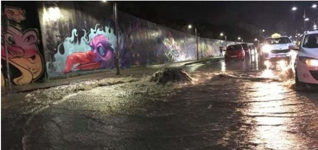
Figure 13. The over flowing sewerage system manhole in Mat neighborhood.
