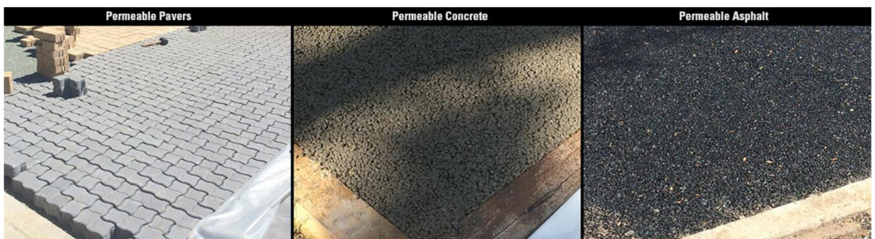
Figure 4 Installations of the three test pavement types: permeable pavers, permeable concrete, and permeable asphalt ( Upper Midwest Water Science Center , 2019)
