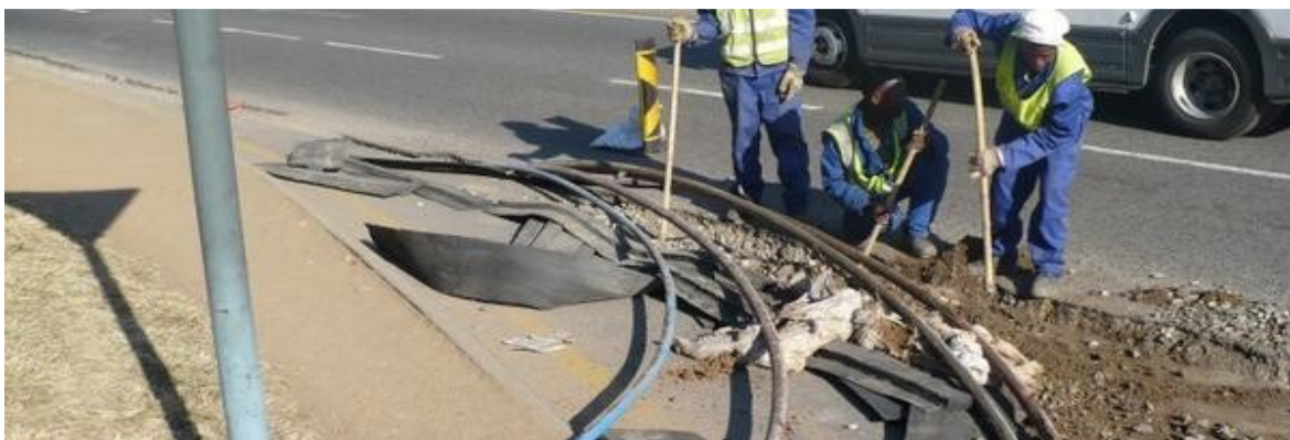
Figure 15 - Rolling out a fiber optic cable in Rwanda
