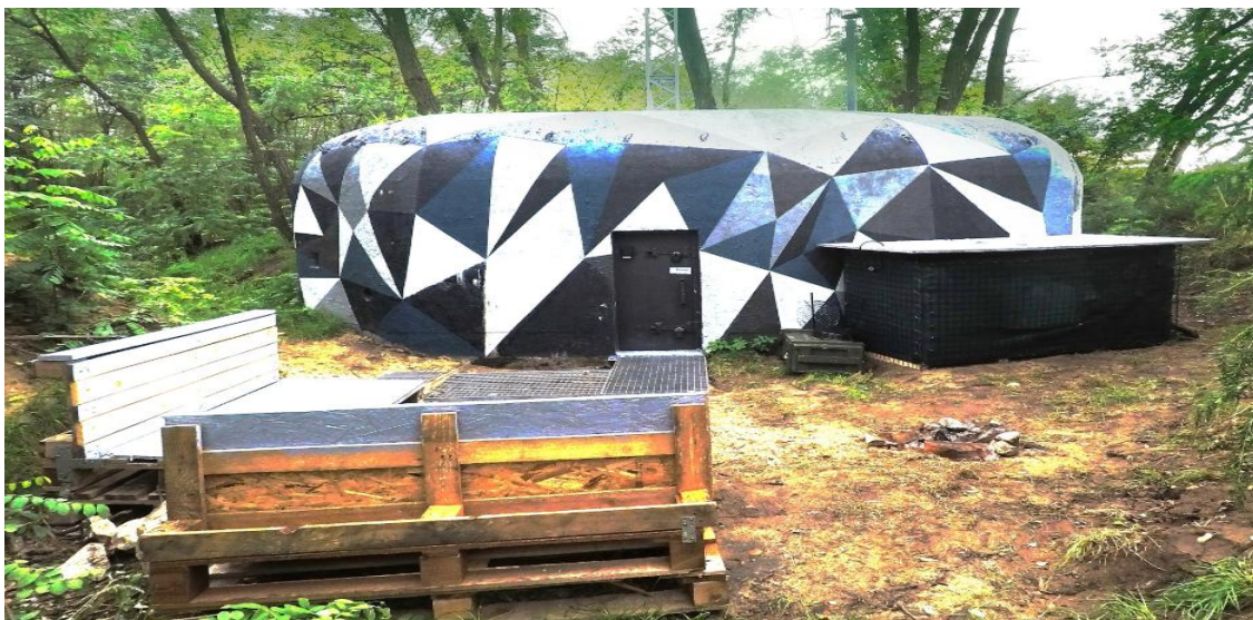
Obrázek 31: Objekt 4/3072/A-160S – Bunkering (BUNKERING.CZ, ©2025)
