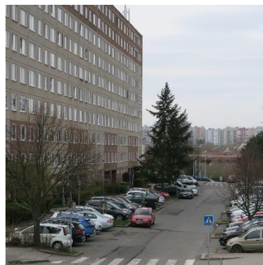
Figure 34- 1980s original modernist block architecture. (Credits: Alisa Malakhova)
