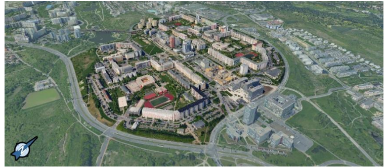
Figure 5- Aerial view. southwest to northeast. (Mapy.Cz, 2023)
