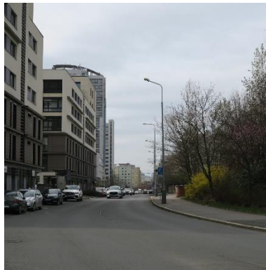
Figure 25- Petržilkova Street condition. Central through street. (Credits: Alisa Malakhova)
