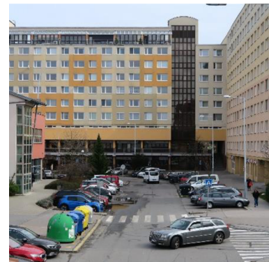
Figure 26- V Hurkah Street condition. South neighborhood part. (Credits: Alisa Malakhova)
