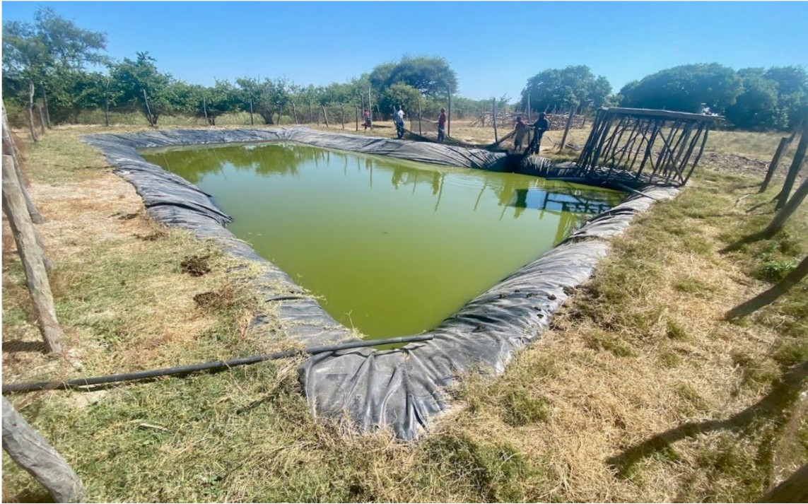
Figure 7. Built dam liner pond in Western Province as part of the Integrated Farming II project (Holistic Solutions 2022)
