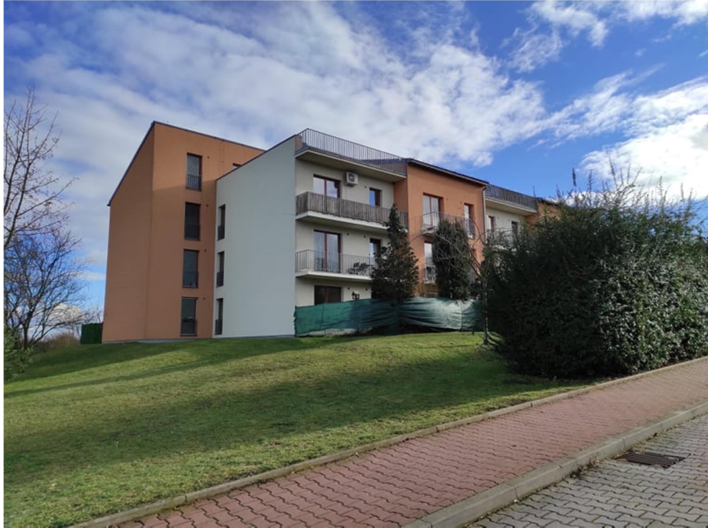
Figure 3.35: Three-story modern architectural building - B. Němcové street, 2021
