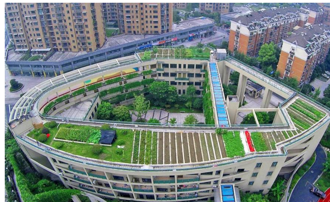
Obr. 13 - Pujia Primary School (Wang, 2015)
