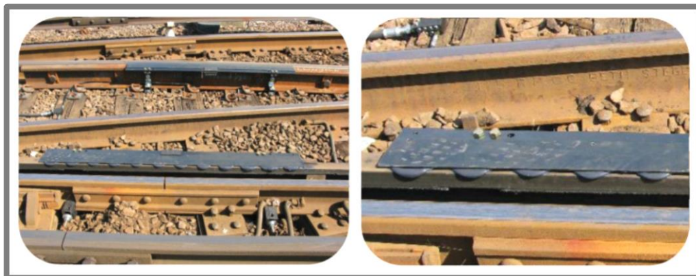
Obr. 3-21 Restraining rail systems [39]
