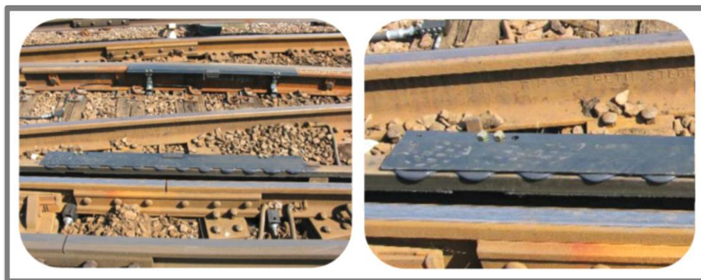
Obr. 3-21 Restraining rail systems [39]
