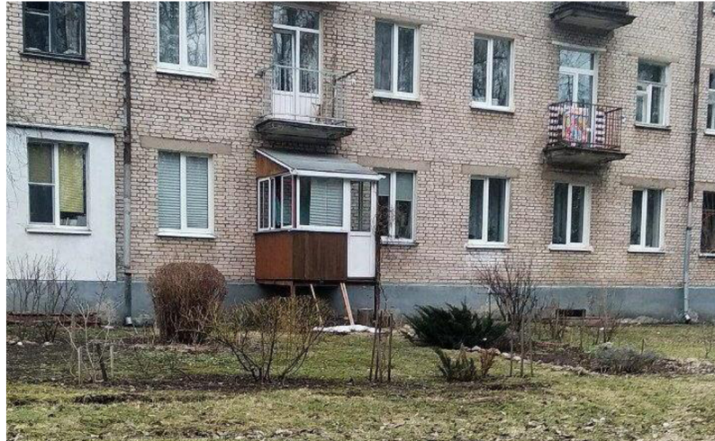
Figure 3.3.5 An example of combined intervention in semi-private space in a post-communist low-story residential area: first-floor glassed balcony extension and land occupation in a form of apartment terrace (Credits: author, Minsk, 2021)
