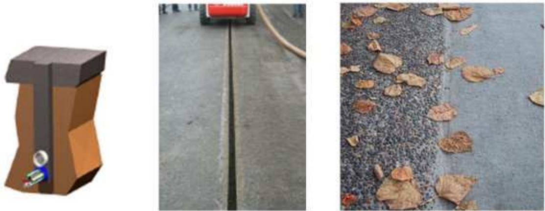
Figure 30: Installation in micro-trenches
