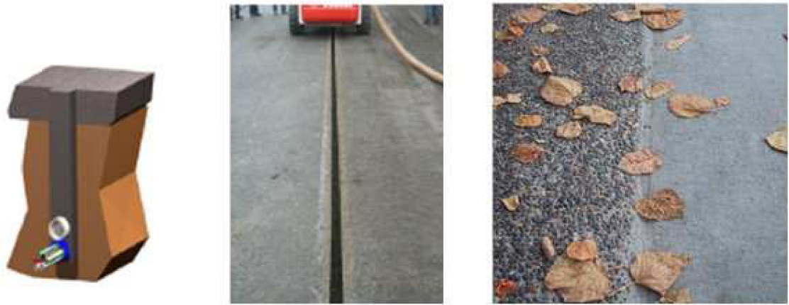
Figure 30: Installation in micro-trenches
