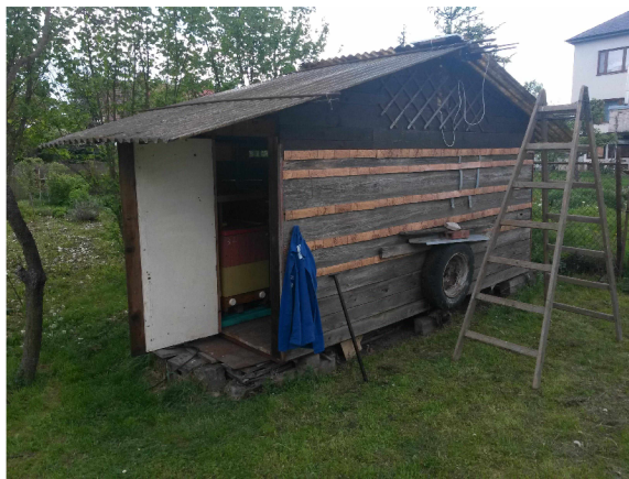
Figure 5.1: Housing of the beehives with mounted solar panel on the roof.
