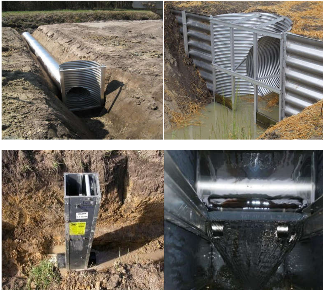
Figure 2: Installation of water control structure
