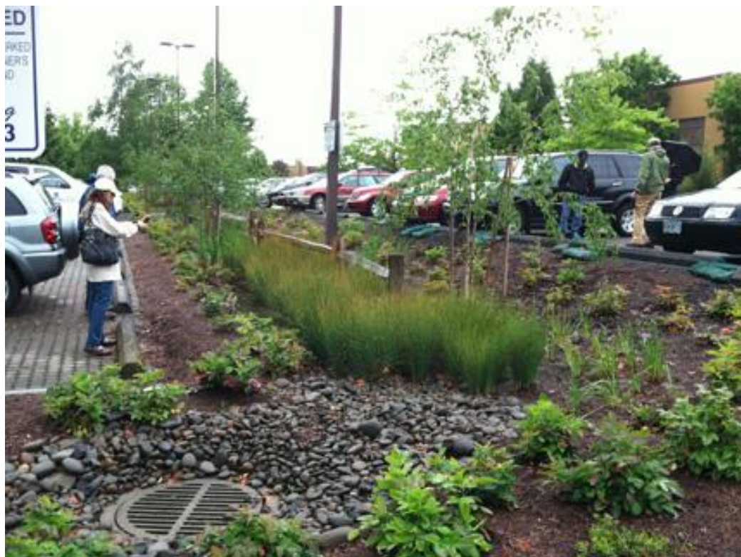
Obr. 7 – Bioswale u parkoviště, Portland, USA (CLEMSON UNIVERSITY, 2017)
