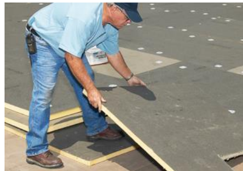
Obr. č. 22 - Instalace tepelné izolace ( http://www.lunaassoc.com/product-lines/commercial-roofing-products/#roof_insulation )
