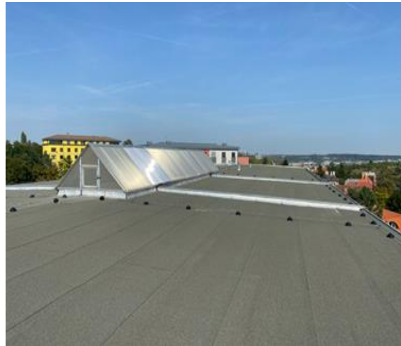
Figure 30 View of the roof where there is great potential for the location of a photovoltaic power plant.
