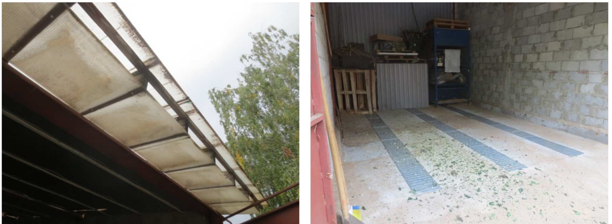
Figure 4.5: Detail of the roof, helio-collector - left; Drying chambre - right (foto: author)
