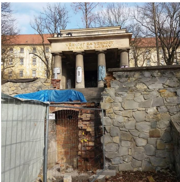
Picture 3: Jihoslovanské Mauzoleum under restoration.
