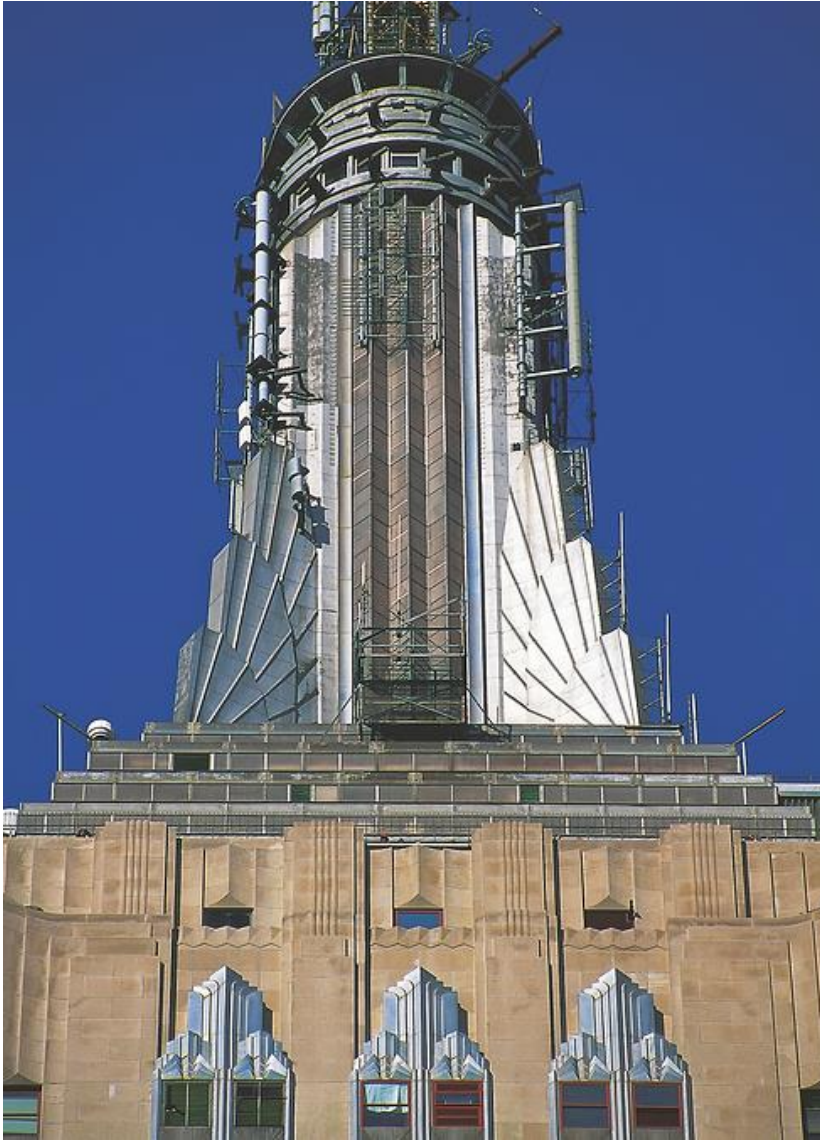
Figure 7: Detailed view of the metal spire at the top of the Empire State Building (Tauranac, 2016).
