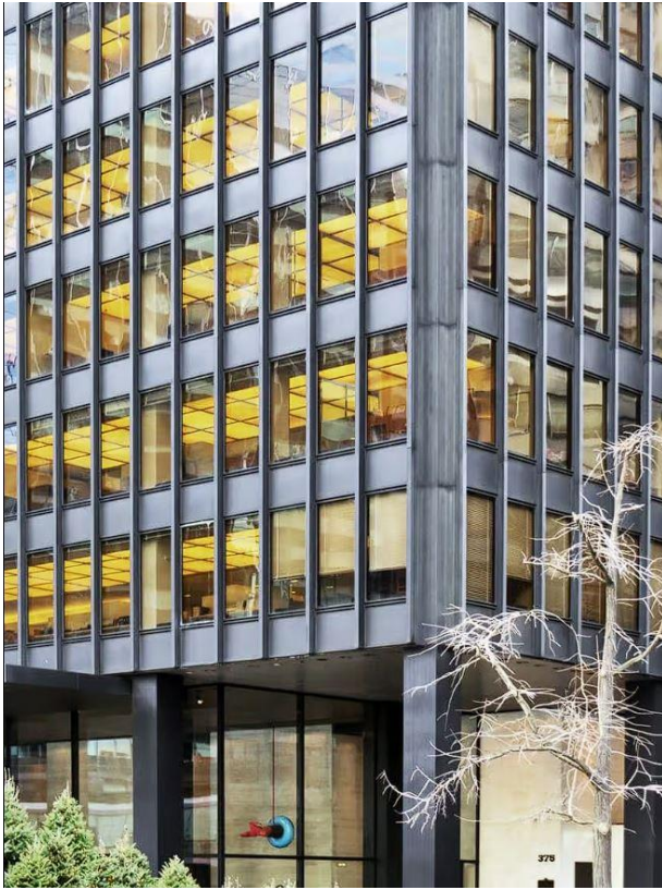
Figure 17: Façade of the Seagram Building in detail (Art In Context, 2022).
