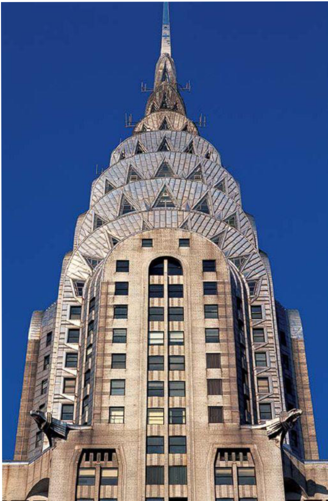
Figure 2: Nirosta crown of the Chrysler Building with its seven concentric ribbed steel arches set with triangular windows (Murphy, 2021).
