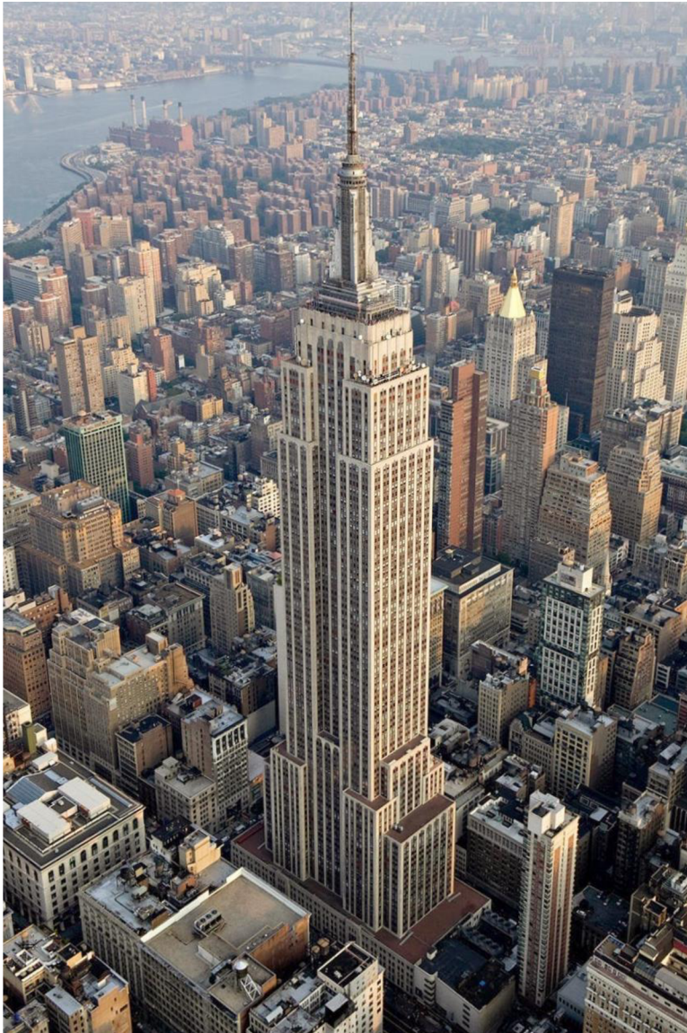
Figure 4: General view of the Empire State Building (Valadi, 2012).
