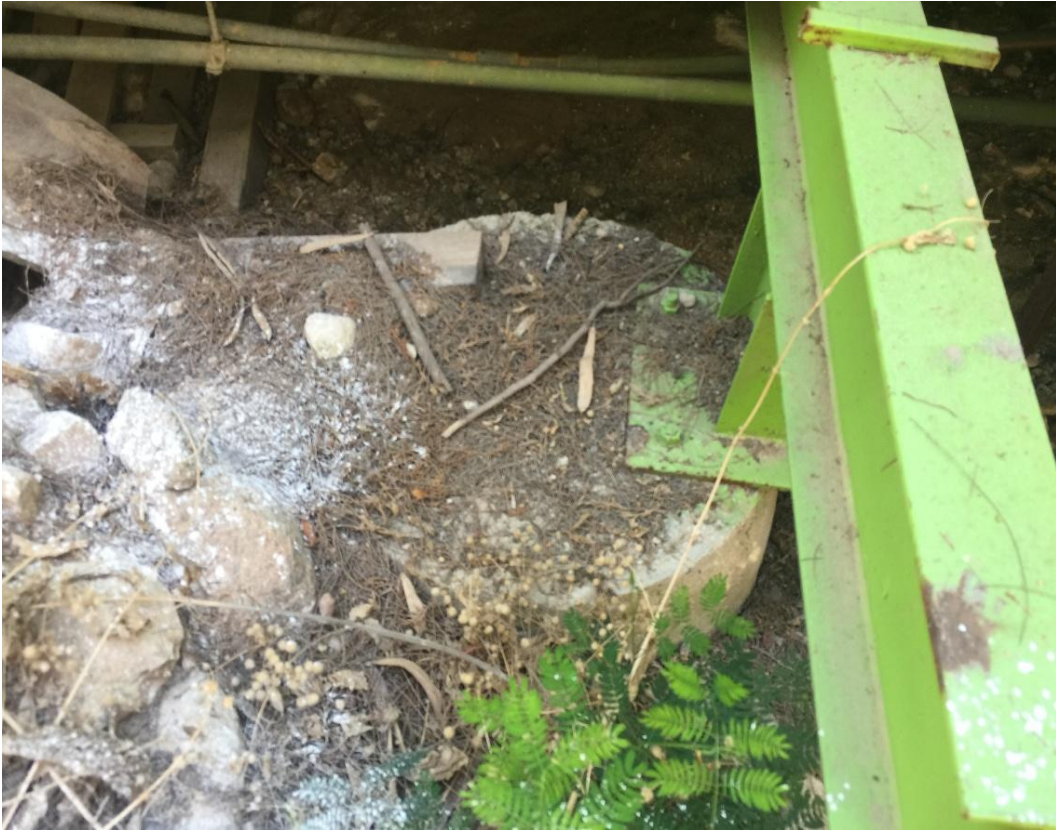
(Figure 6) Abandoned Biogas plant in ALGhoor region.
