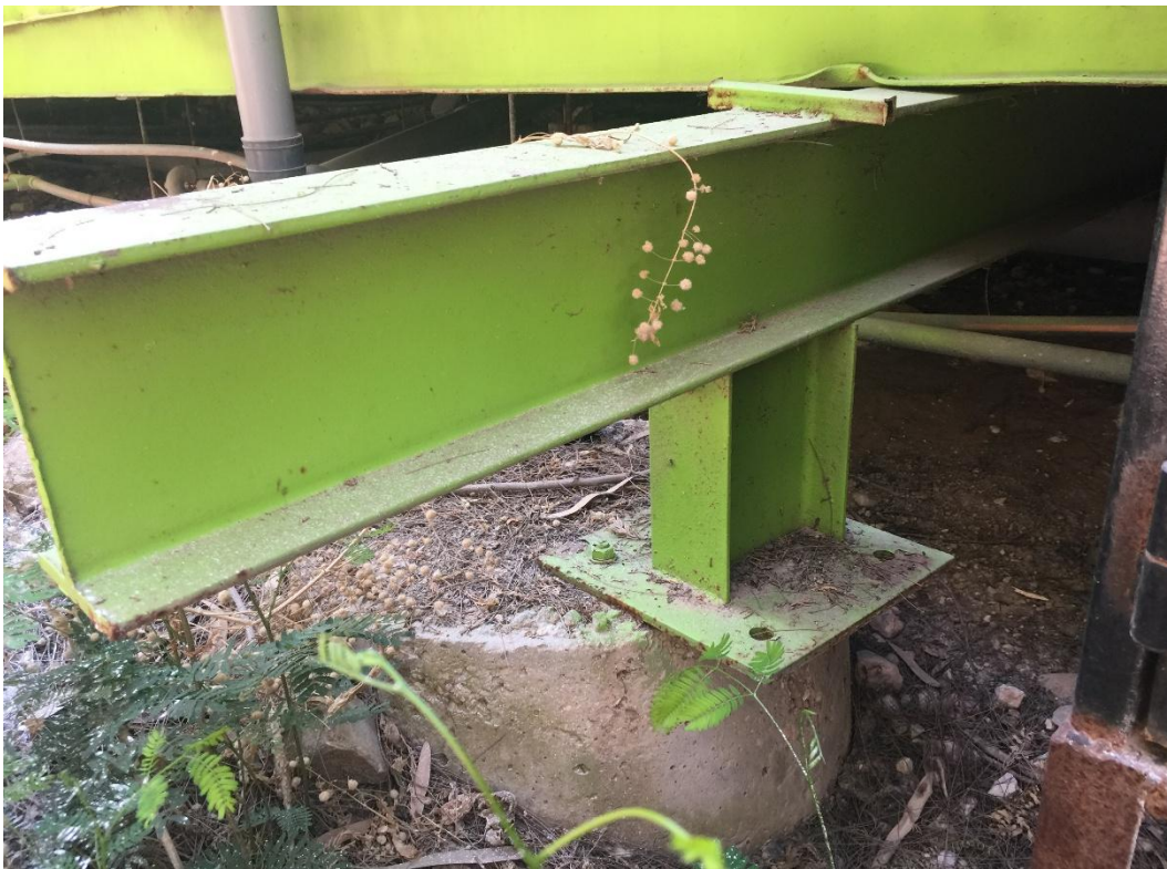
Abandoned Biogas plant in AlGhoor region.
