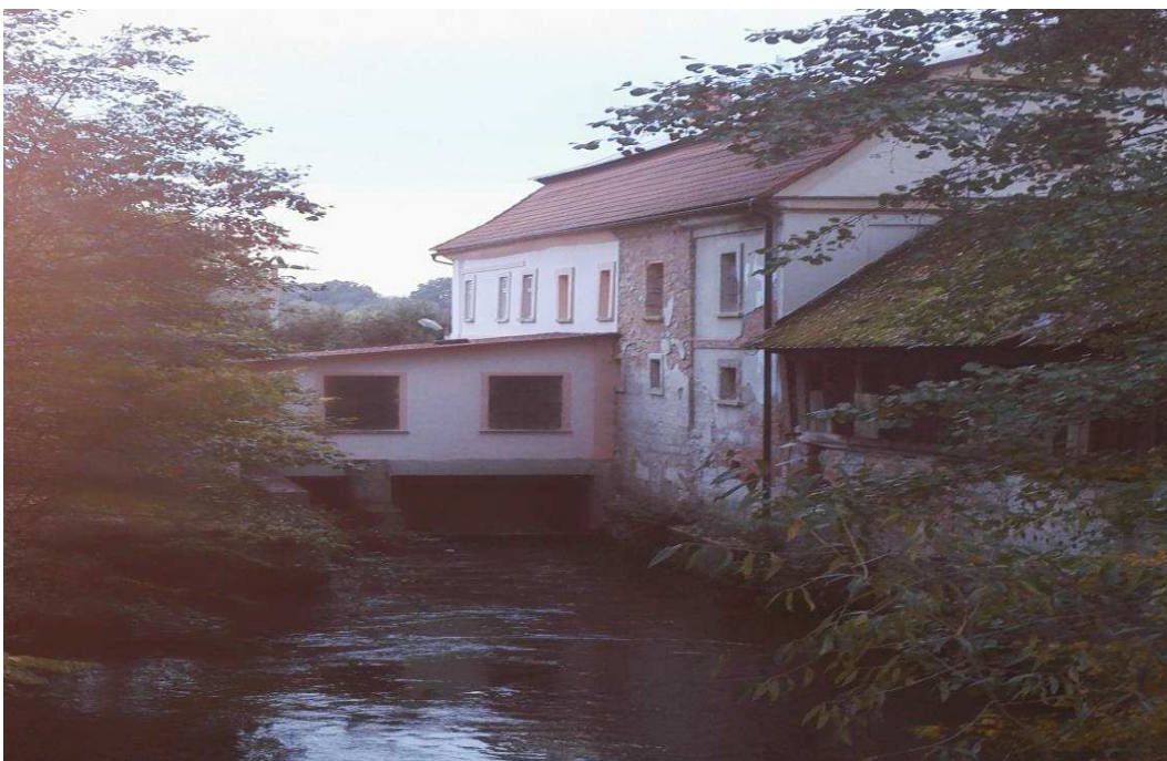
Obr.44 MVE Stanovice I
