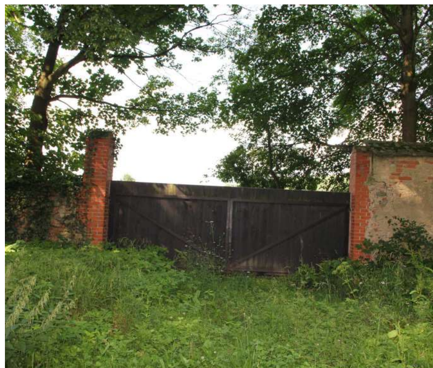
Obr. 37. Technický vjezd nad terasami
