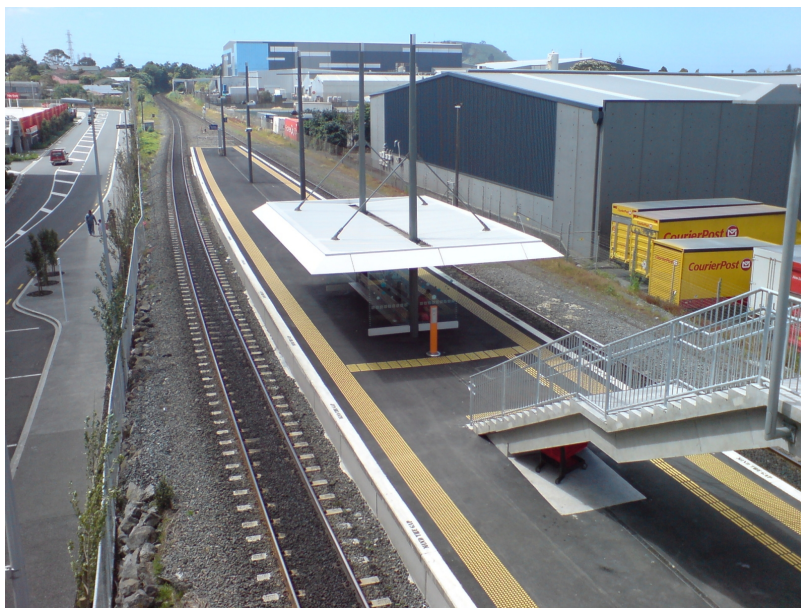
Figure 2.1: Tactile pavement in Sylvia Park New Train Station (yellow color) [10]
