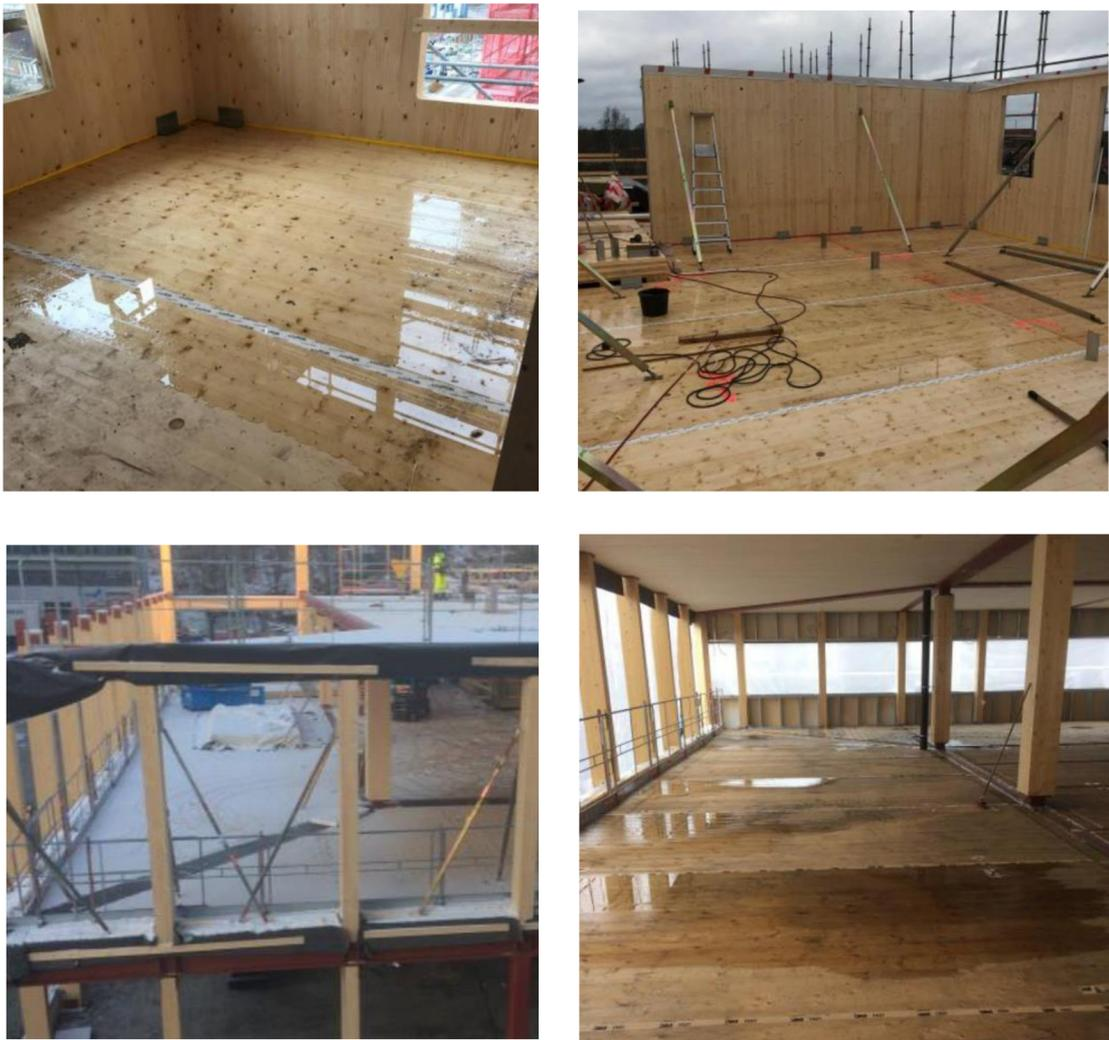
*Figure 27 - CLT panel ceiling exposed to pooled water (Olsson, 2020)*
