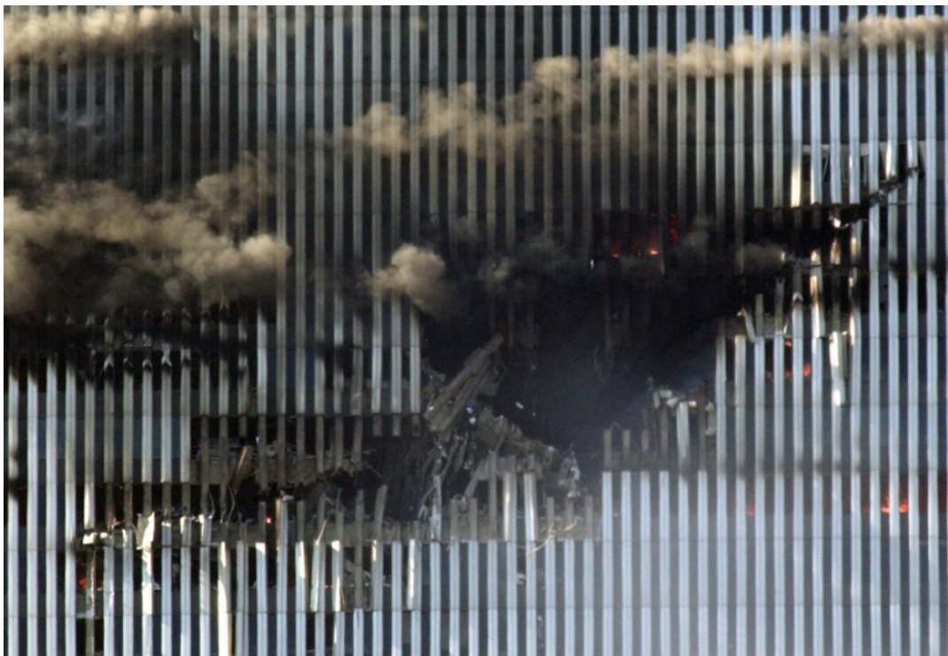
Figure 16: Hole from Flight 11 in the North Tower, 33 Page 15
