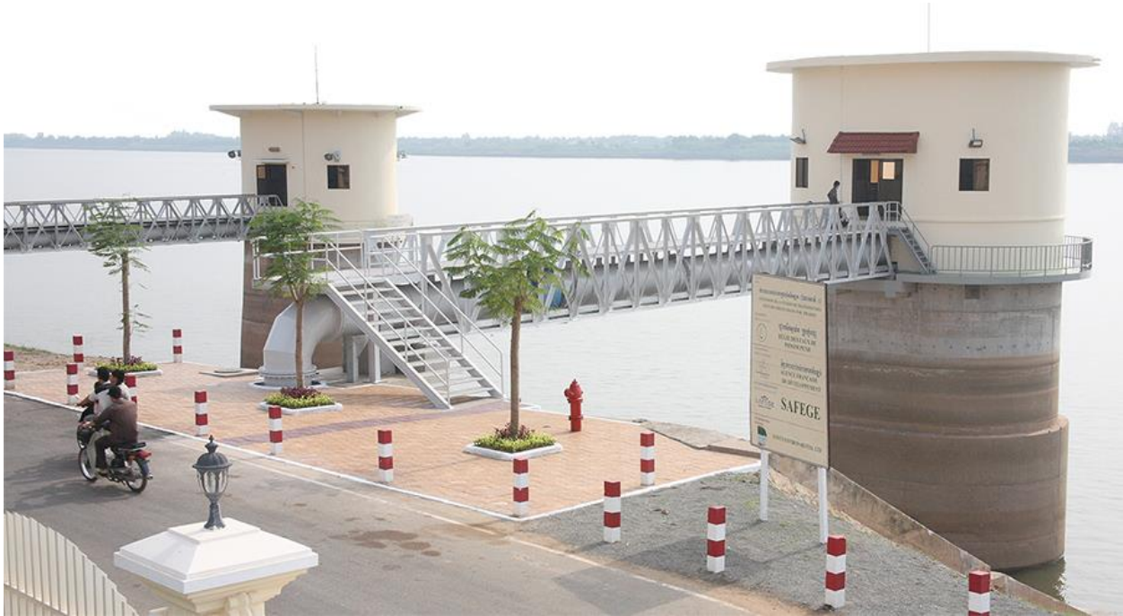
Figure 8 Water intake tower in Phnom Penh
