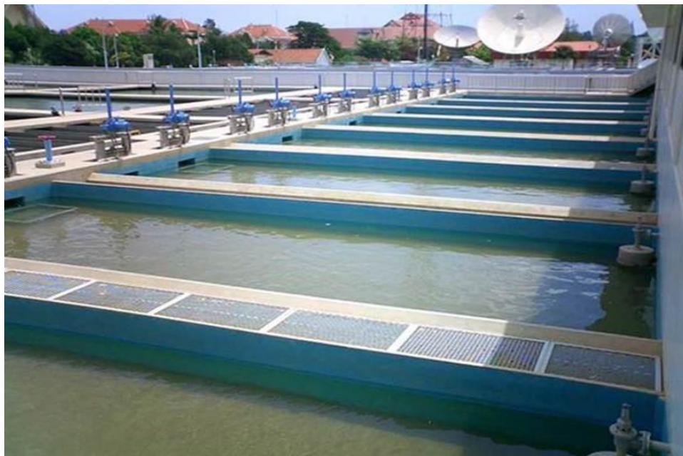
Figure 12 Filtration tank
