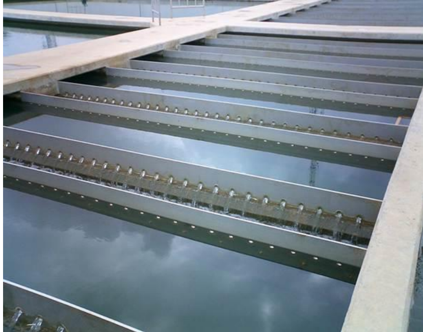
Figure 13 Sedimentation tank
