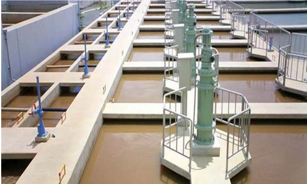
Figure 11 Flocculator tank
