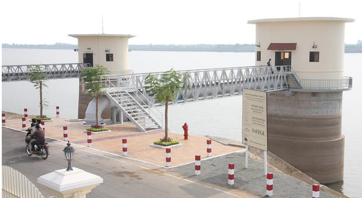
Figure 8 Water intake tower in Phnom Penh
