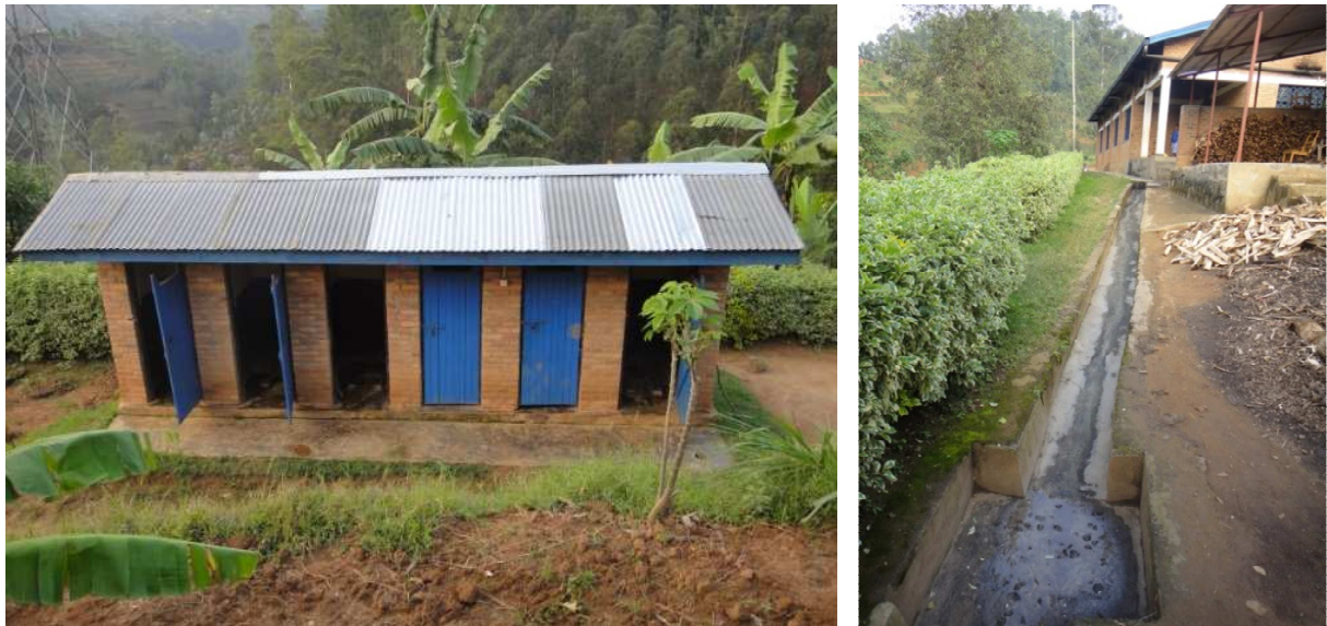
Figure 7: Pit Latrines (left) and storm water gully at Future for Kids (right) (own pictures, 2014)
