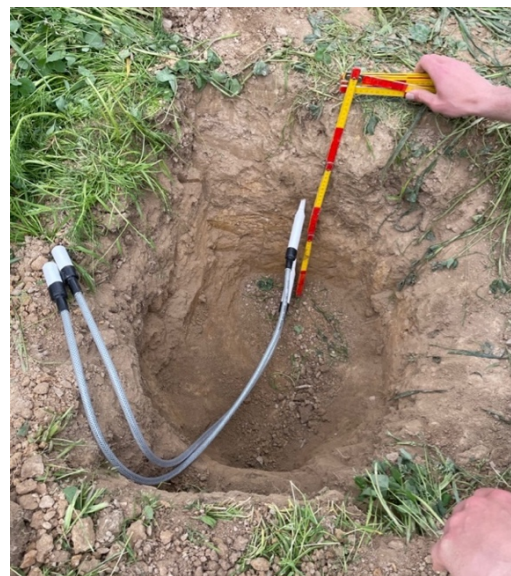
Fig. 23: Installed 25 cm and 50 cm TMS monitors
