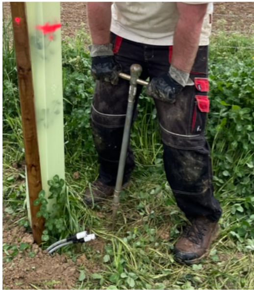
Fig. 24: Metal tool being wedged into the soil with a driving device
