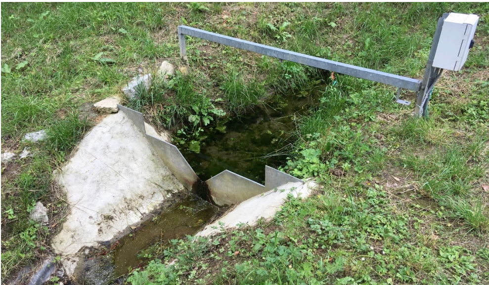
Picture 1: Detail of the drainage (bottom) and sedimentation pond with a distribution box from where the water is distributed to the constructed wetlands (top). Photo Jan Vymazal
