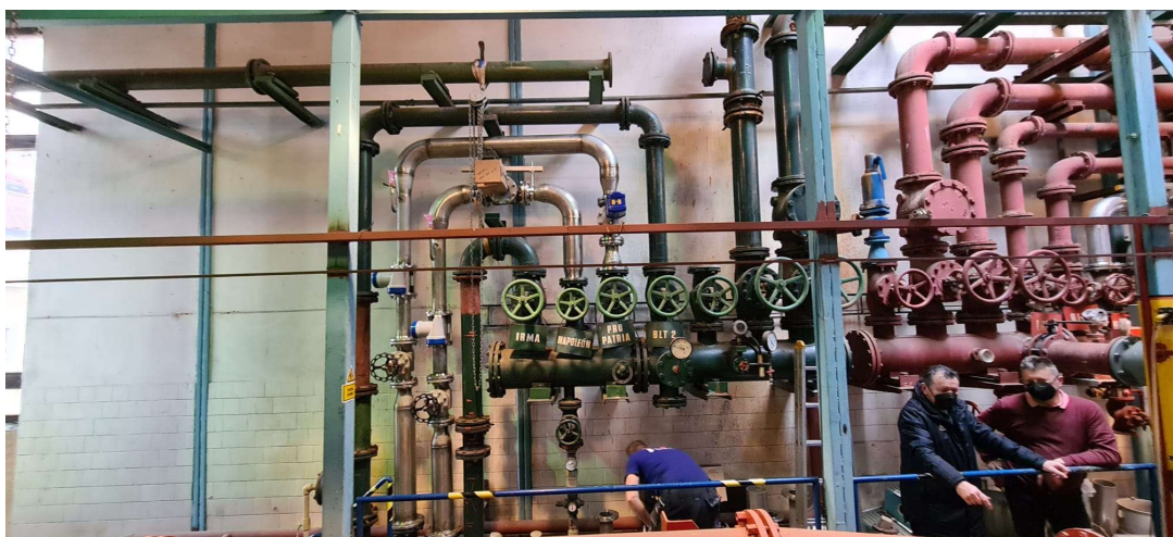
Picture 4.32. Revitalization of distribution system for natural healing water
