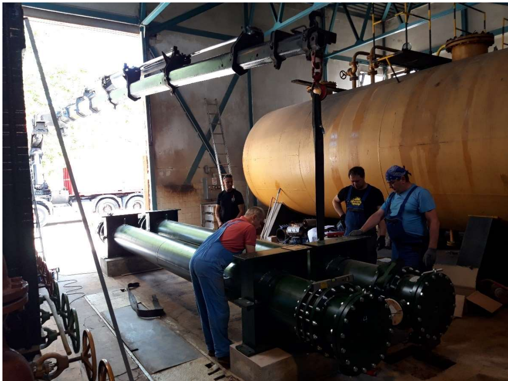
Picture 4.30. Assembling of new graphite heat exchanger
