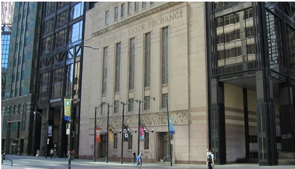
Figure No. 9: “Toronto Stock Exchange” building
