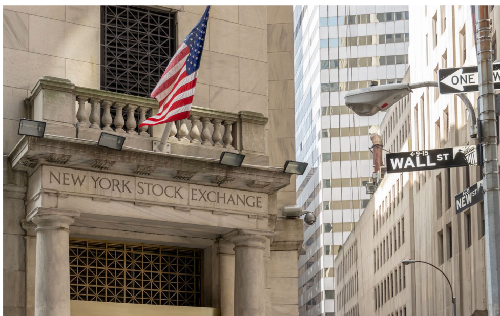
Figure No. 1: “New York Stock Exchange” building
