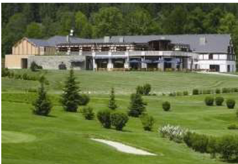
Obr. 6: Objekt hotelu Golf Cihelny
